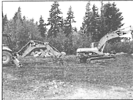
Photograph 7: Placing backfill in SPN. View looking north.
